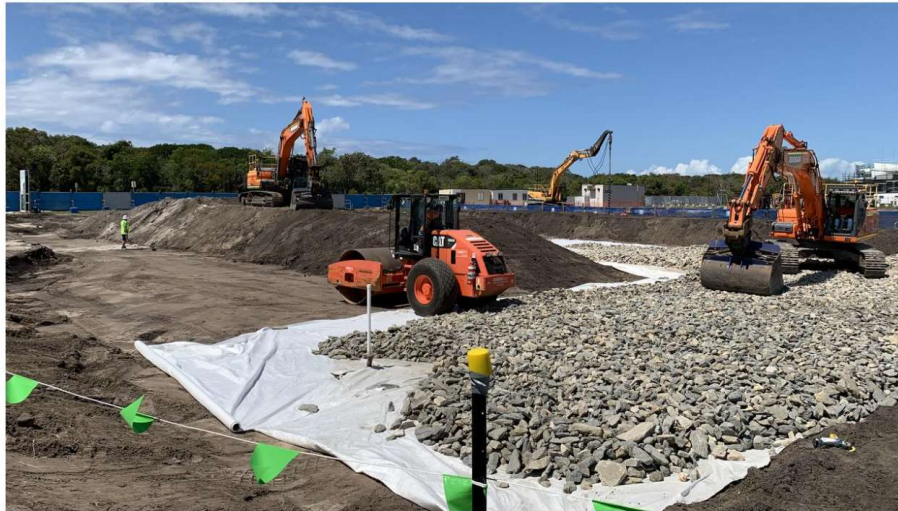
UNDERWAY: The Seanna Residences at Bokarina Beach are underway.
